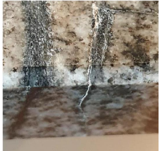
Close-up of a leading edge and the underside of the worktop, showing a through-crack with a visible gap between the fracture surfaces.
