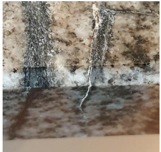
This is a close-up image of a leading edge. Note that there are gaps in the crack and that it is continuous through the thickness of the slab.
