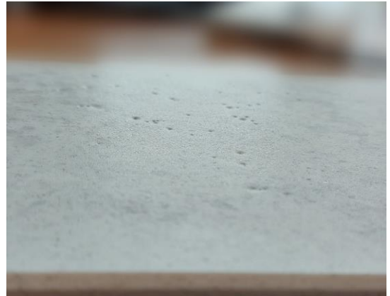
Example of a concentration of pinholes that is not acceptable and is grounds for complaint
